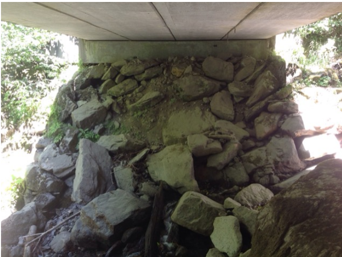
Right Bank Abutment when facing downstream
