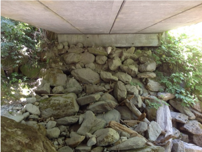
Left Bank Abutment when facing downstream
